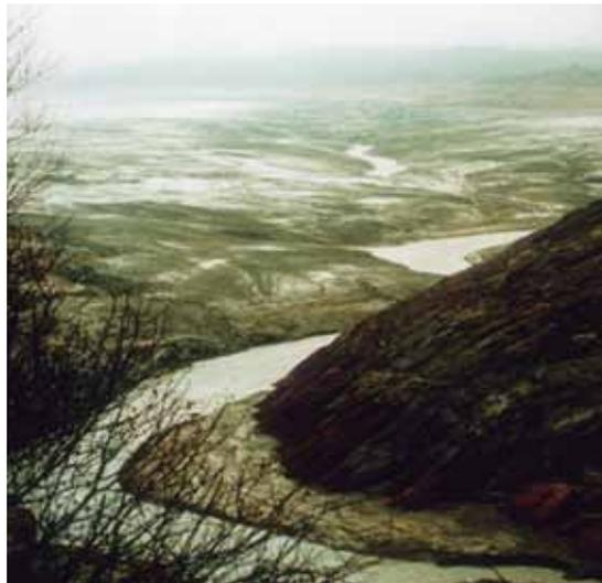
**Figure 6.** Upstream view from the Joaquín Costa dam in 1995, just after the reservoir was emptied through the bottom outlets to release part of the sediments. Two thirds of the sediments remained in the reservoir. Image R.M. Poch.
